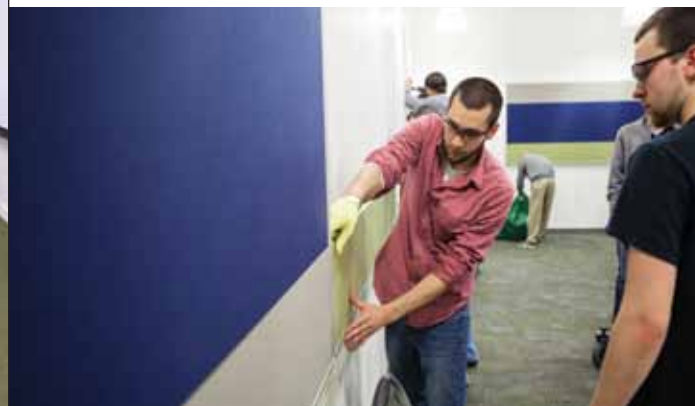
Students installing Ecophon® Texona™ Wall Panels
